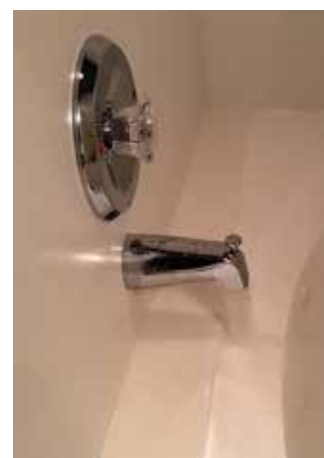
Figure 3: Basin tap fixed in the wall with no extension pipe for a usable water flow
