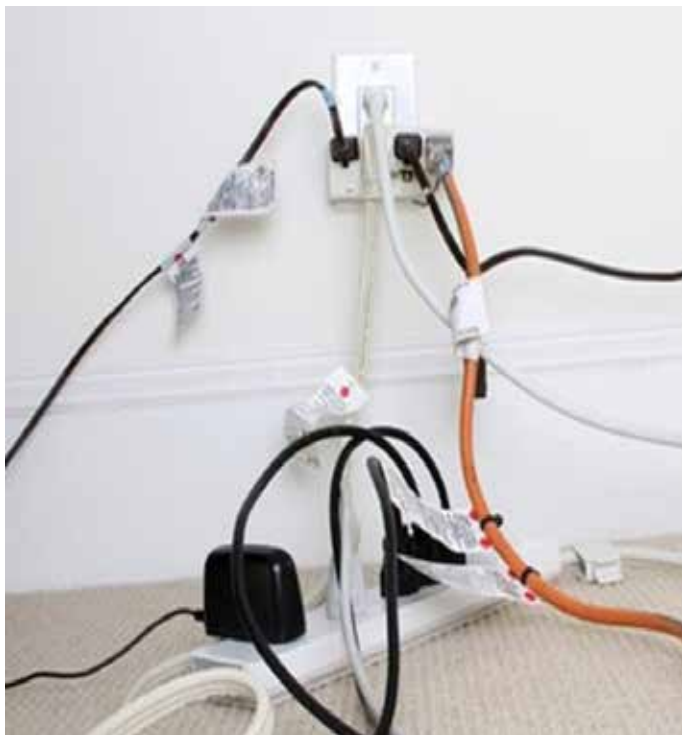
Figure 12: A single plug point with multiple chargers. No provision of sufficient plug points
