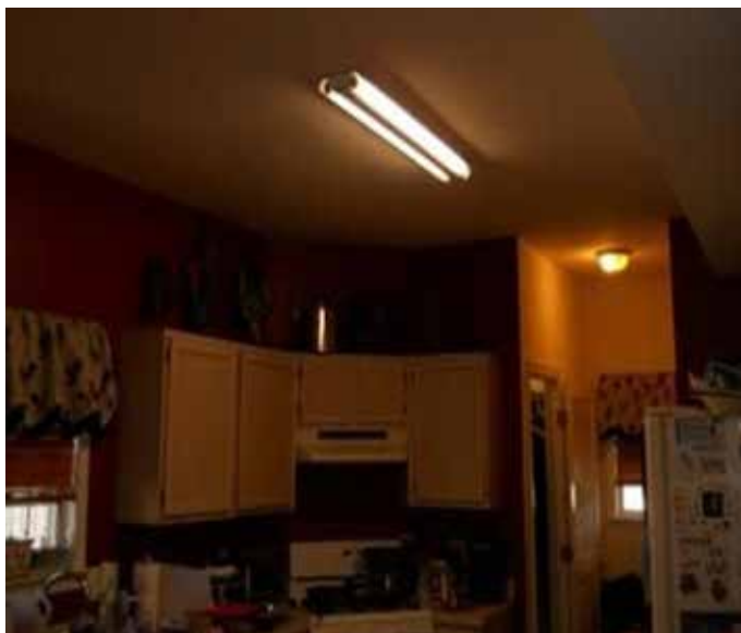
Figure 10: No task light or sufficient light provided in the kitchen to work on the platform
