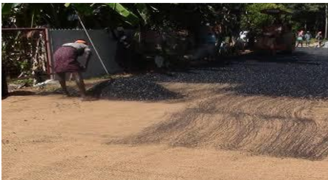
Fig.7 A Road constructed using Coir Fiber in Kerala
